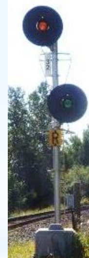
Intermediate signal to Sunalta looking east.
