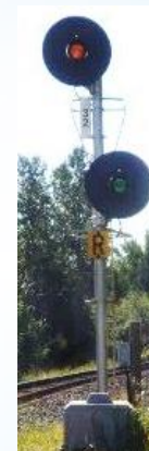
Intermediate signal to Sunalta looking east.
