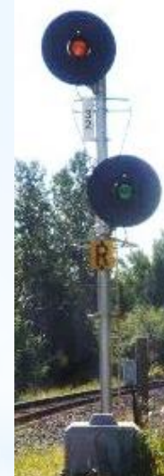
Intermediate signal to Sunalta looking east.
